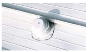
Ballew's Roof-Over System uses a specially formulated tar tape to seal vents against leaks and water damage.
